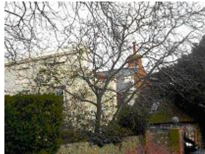
Ovingdean Grange – view from the south-east.
